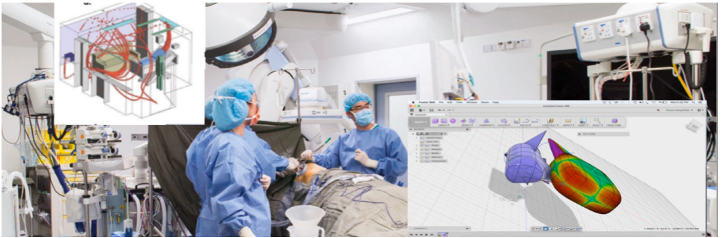
Figure 2 View on a typical surgery environment with computational fluid dynamic test sequences with Autodesk CFD and Fusion 360 / Solid Works of controlled air and ventilation distribution avoiding the spread of pollutants, bacterias and other impacts. Source: Thomas Spiegelhalter, 2016.
